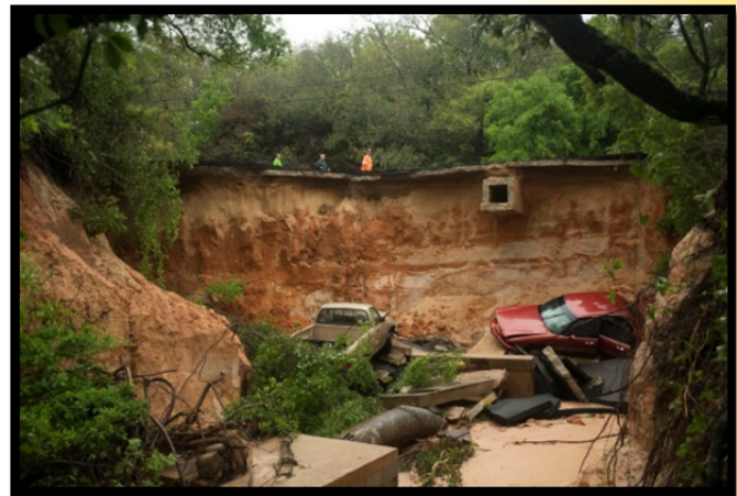
People survey the damage on Scenic Highway after part of the highway collapsed following heavy rains and flash flooding in Escambia County. Source: Reuters, Michael Spooneybarger
