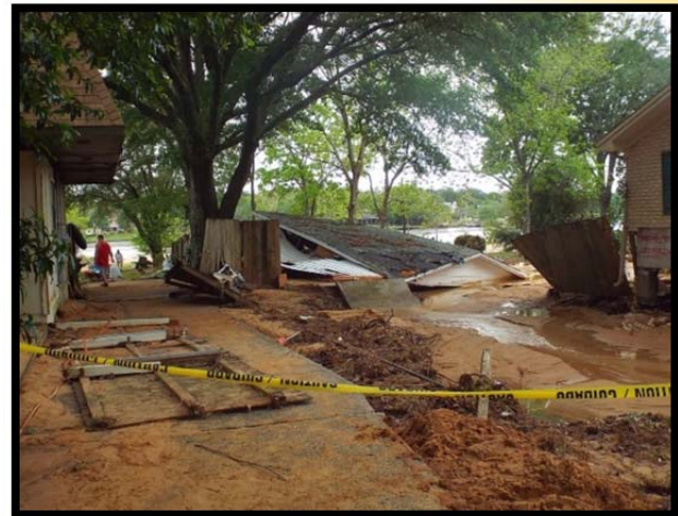
Flood damage in Pensacola, FL. Source: Pensacola News Journal
